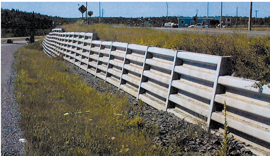
Figure C14. Schematic and photograph of a steel bin wall. (Schematic from Reference 11.)
