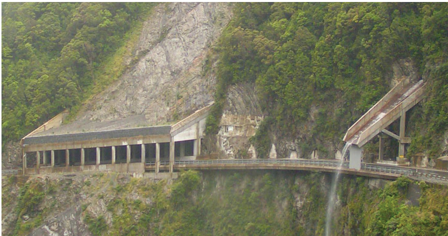
Figure C25. Example of an open rock shed in New Zealand (Photograph courtesy of Richard Wright, rock climber).
