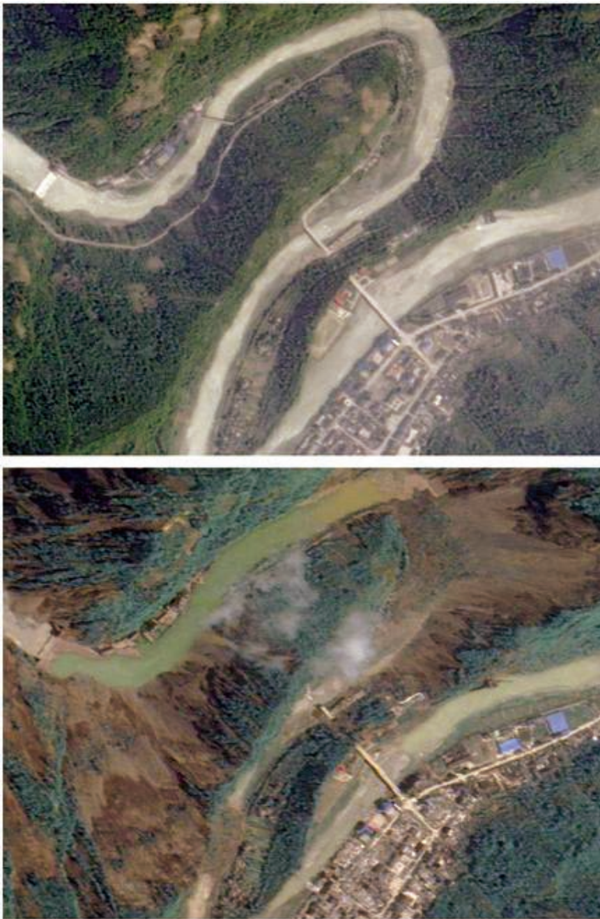
Figure 43. The great earthquake that struck China on May 12, 2008, caused extensive damage in the mountainous terrain of Beichuan County. In many cases, landslides in steep valleys formed landslide dams, creating new lakes in a period of hours. This pair of high-resolution, photo-like images from Taiwan’s Formosat-2 satellite on May 14, 2006 (top), and May 14, 2008 (bottom), before and after the earthquake, show the large landslide that blocked the Jiangjian River, forming a dangerous landslide-dammed lake.
