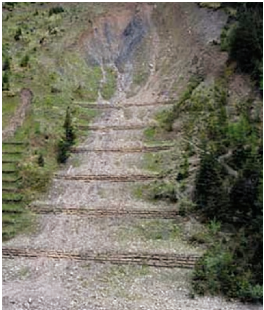
Figure C7. Schematic and photograph of a crib wall check dam, which is one kind of check dam. (Graphic from Reference 11, photograph taken in Trafoi, Italy, courtesy of "Erosion Control," Forester Communications, Santa Barbara, California, USA.)
