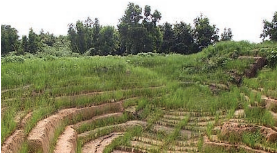
Figure C18. A Vetiver grass system is being used in the Democratic Republic of the Congo for gully control in urban areas and for highway stabilization. These gullies are a major problem in this area and other West African countries ( top ); the same slope now has improved drainage, and the slope has been planted in Vetiver grass ( middle ); this planting of Vetiver grass is about 3 months old ( bottom ).
