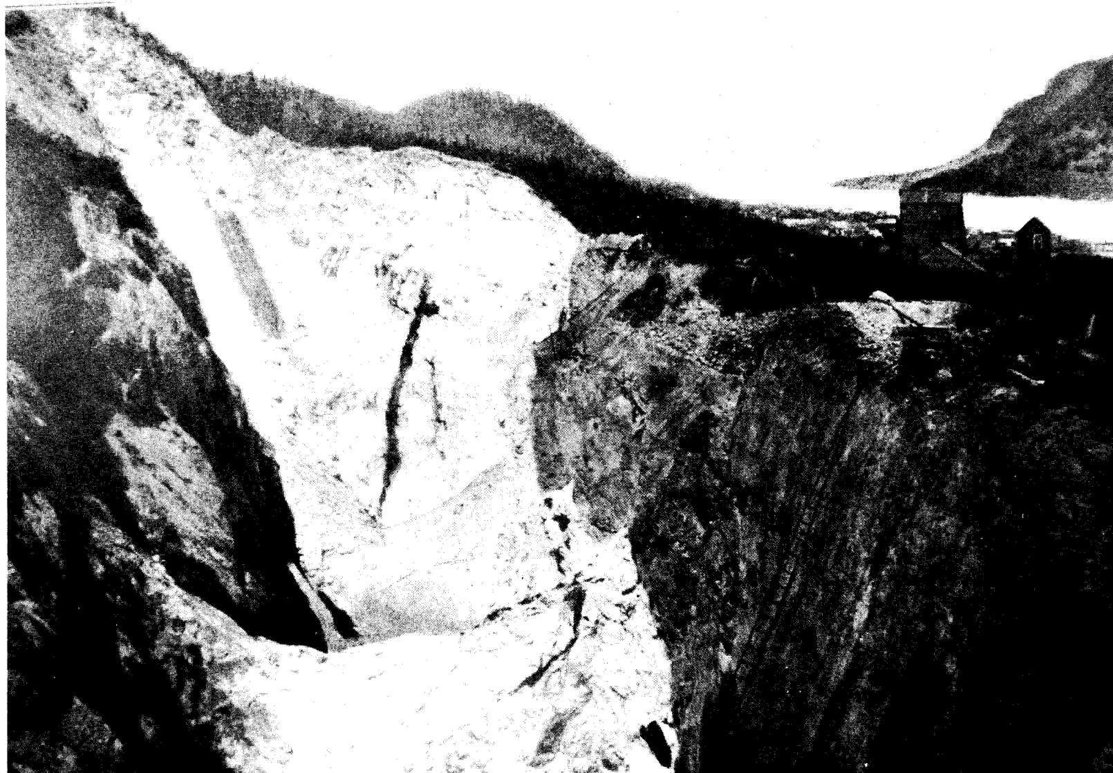
Figure D-31.—The Treadwell sill and orebody, 1904. This light-colored albitized diorite sill was mined to a depth of 2,800 feet and yielded 3.2 million ounces of gold (photo from Spencer D-130 ).
