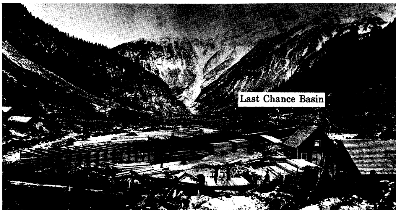
Figure D-120.—The Jualpa Placer Mine, Last Chance Basin. Although extensive work was done to develop the placer, problems including large boulders, tree stumps, and floods, precluded any significant gold recovery (photo courtesy Alaska State Library, Winter & Pond collection).
