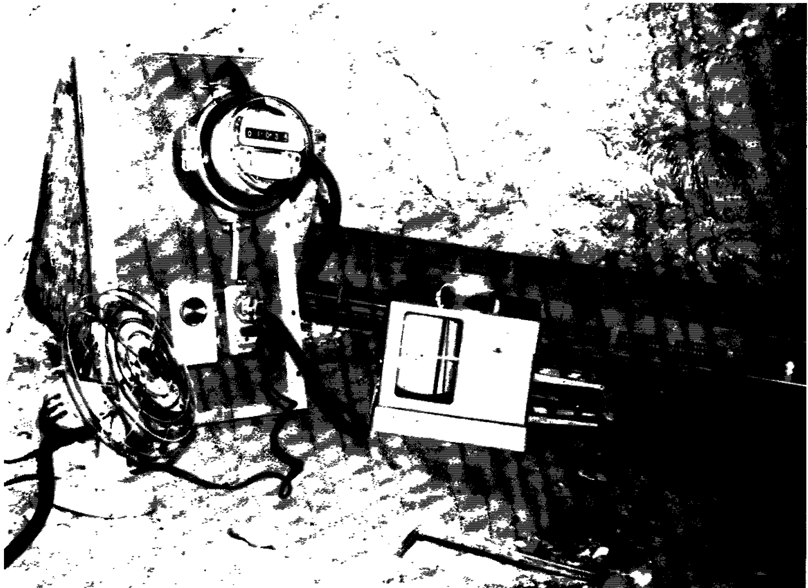
FIGURE 16. - Heating and Monitoring Equipment Inside Foamed Room.
