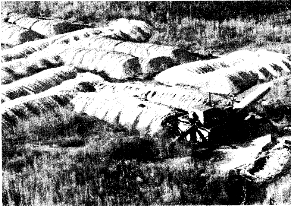
FIGURE 2.—Dredge on Woodchopper Creek.
