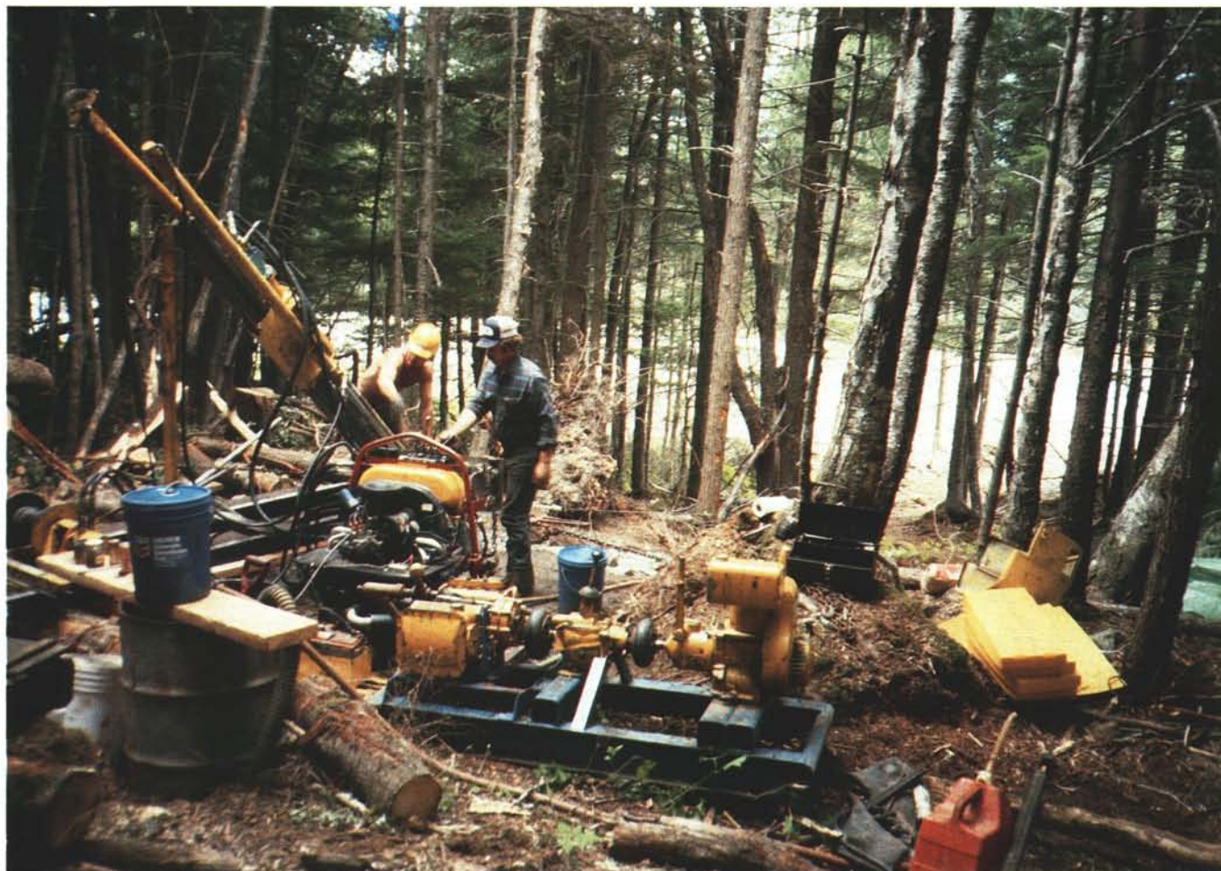
Bureau drilling at the Road Cut prospect (Haines-Klukwan-Porcupine subarea).
