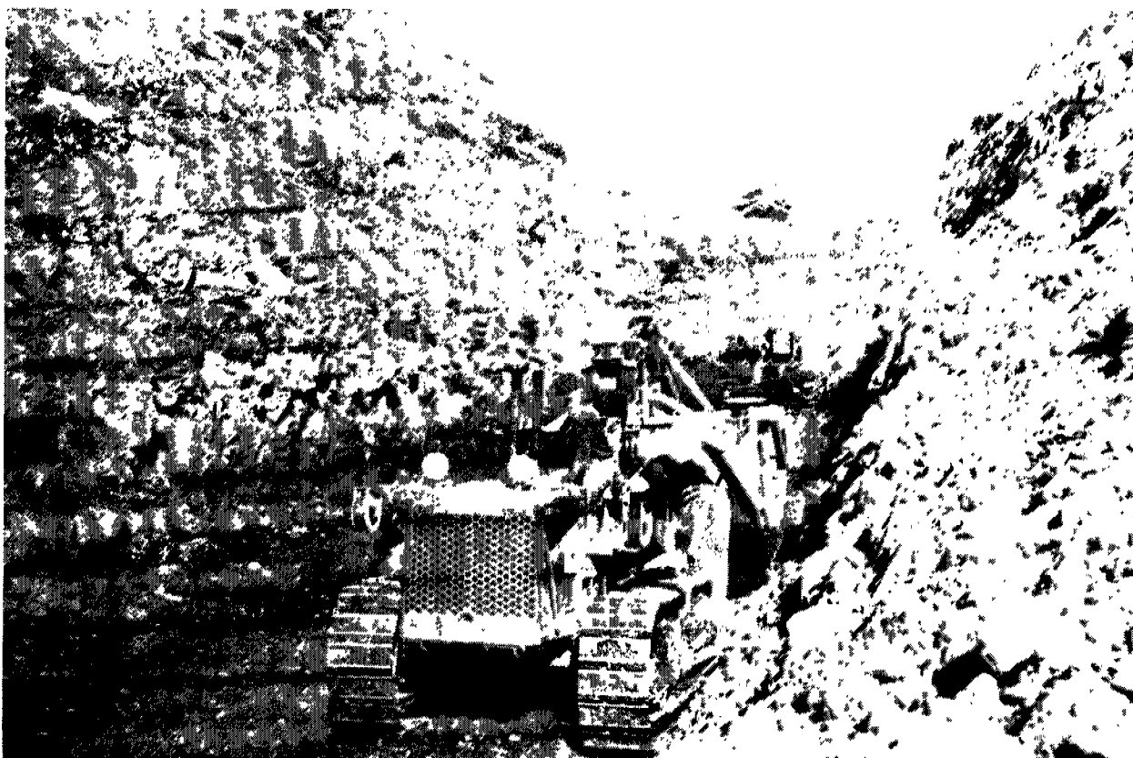
FIGURE 4. - Skull Creek Fire Area in Colorado, Showing Equipment Working in Isolation Trench.
