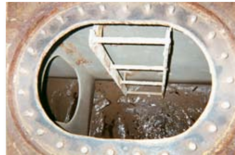
Ballast water and sediment residuals in ballast tanks.
