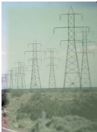
Getting power from generating facilities to the public is a challenge
