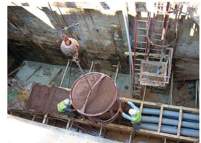
Katy Freeway Duct Bank Relocation.
