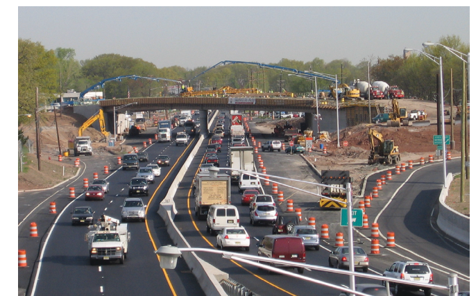
New Jersey Route 17 – Essex Street Bridge Reconstruction.
