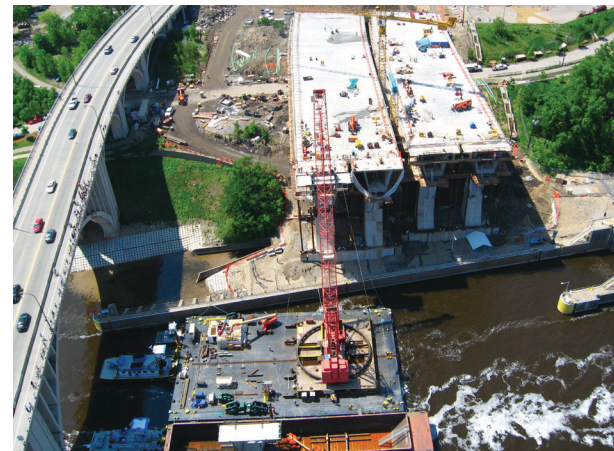
I-35W Bridge Replacement.
