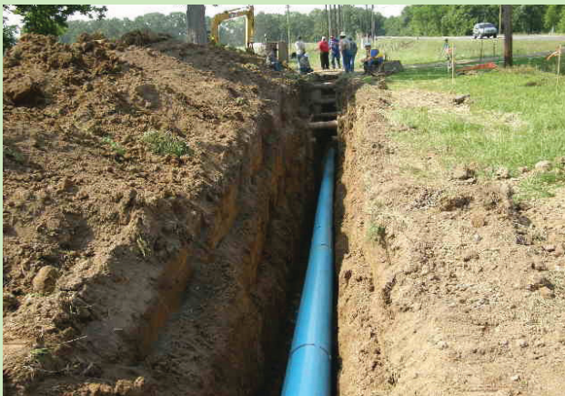
Ambassador Caffery Parkway Utility Relocation.
