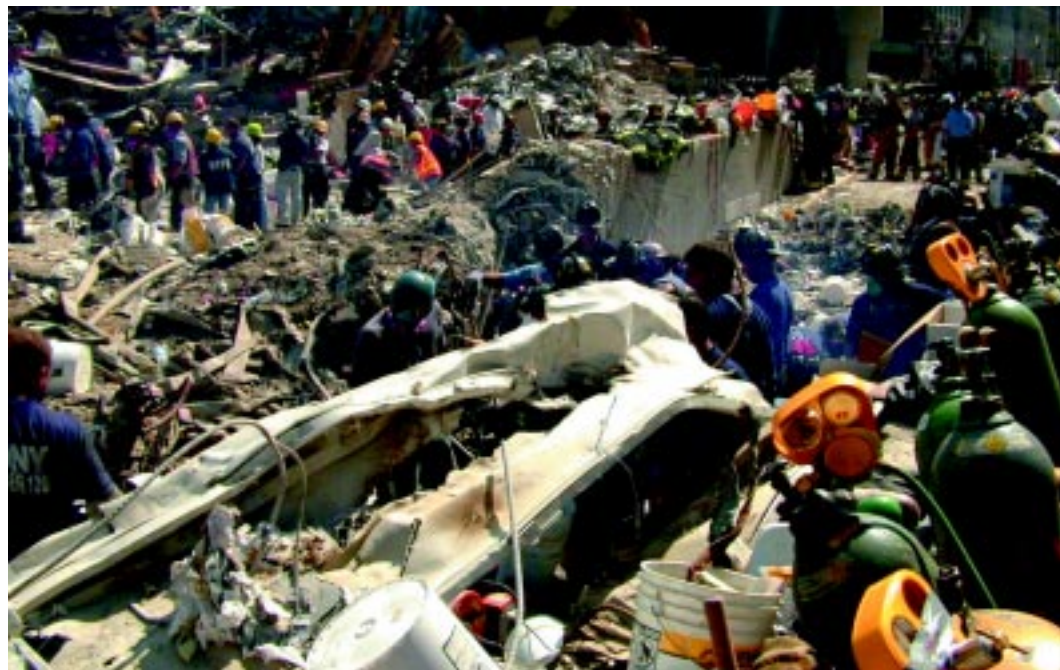
Hundreds of rescue workers and firefighters sift through rubble near the building that once housed OSHA’s Manhattan Area Office. FEMA photo by Michael Rieger
