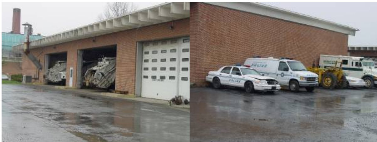
Figure 3-3. Photograph of the drainage area.
