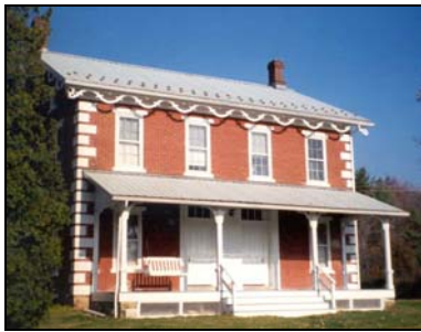
Arney House, Centre Hall, Potter Township, Centre County. Four-over four, two-door house.
