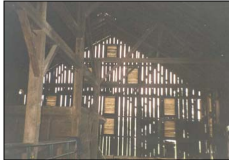
Taylor Potter barn, Potter Township, Centre County, interior of straw shed. Note the centrally located granary.
