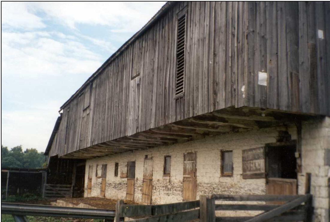
Neubert barn, Rimmey Road, Centre County. Forebay side. Notice doorways to feed aisles and animal pens. This example has a machinery storage bay incorporated into the lower level.
