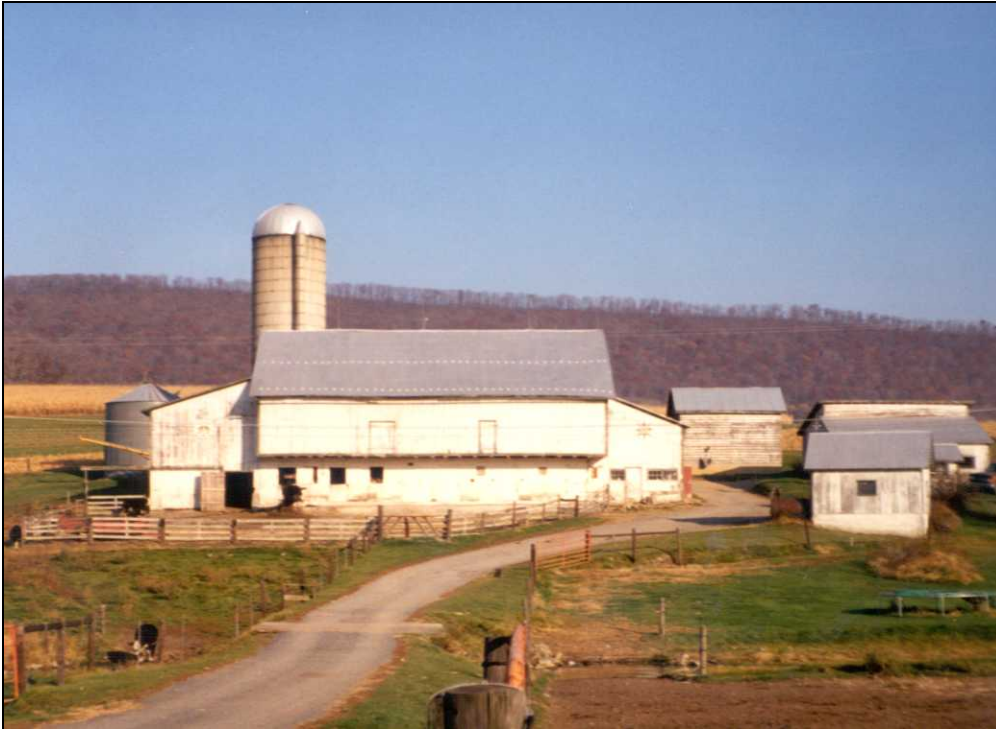
Pennsylvania Barn, Linden Hall Road, Harris Township, Penn's Valley, Centre County.
