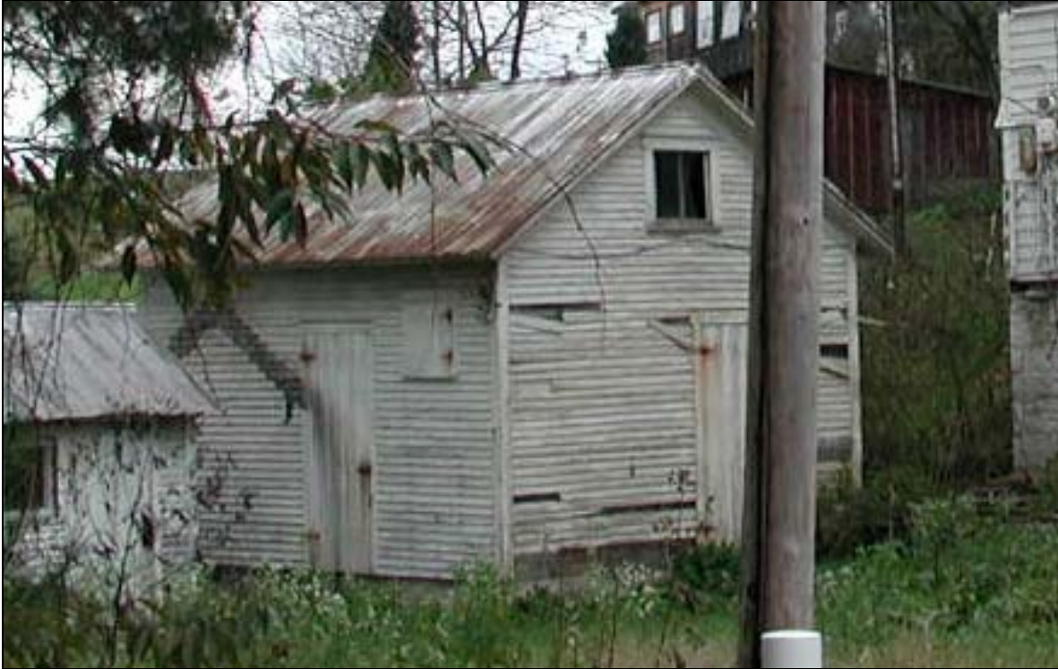
Long Lane, Centre County. This outbuilding has the blank walls and raised foundation that might suggest an ice house.
