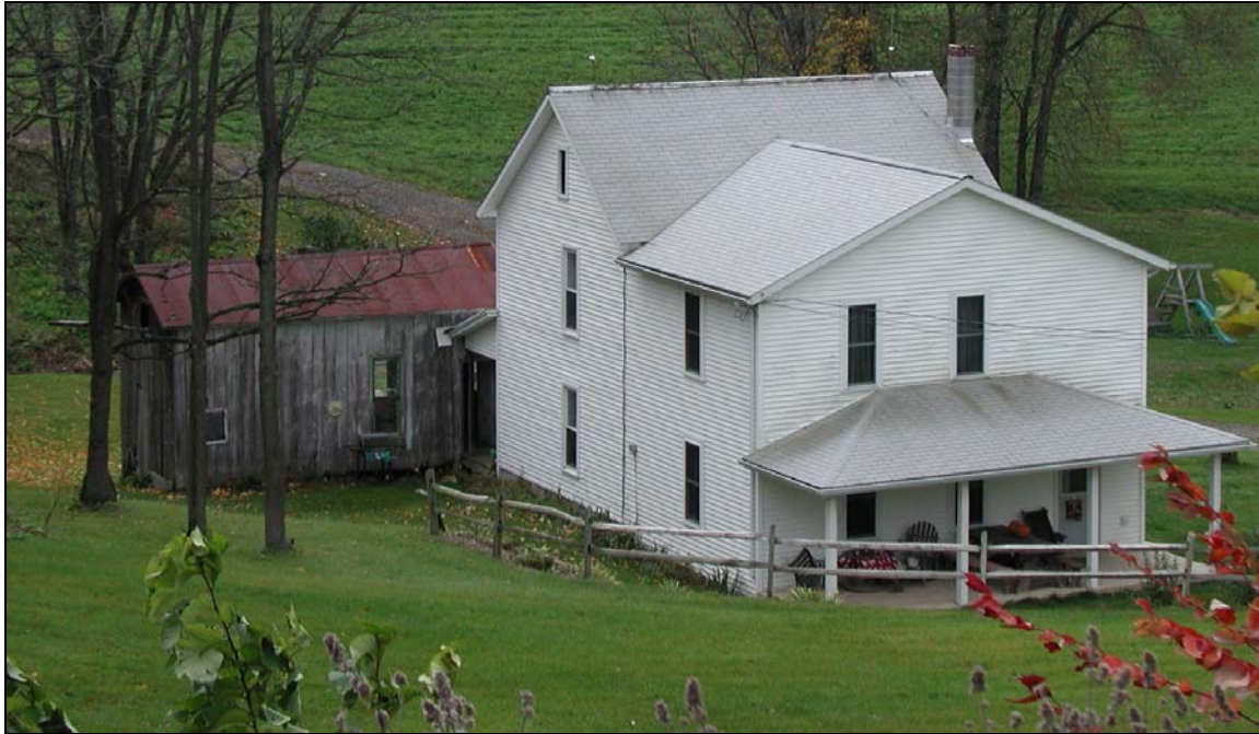
Summer kitchen and house, Heckman Cemetery Road, Centre County.
