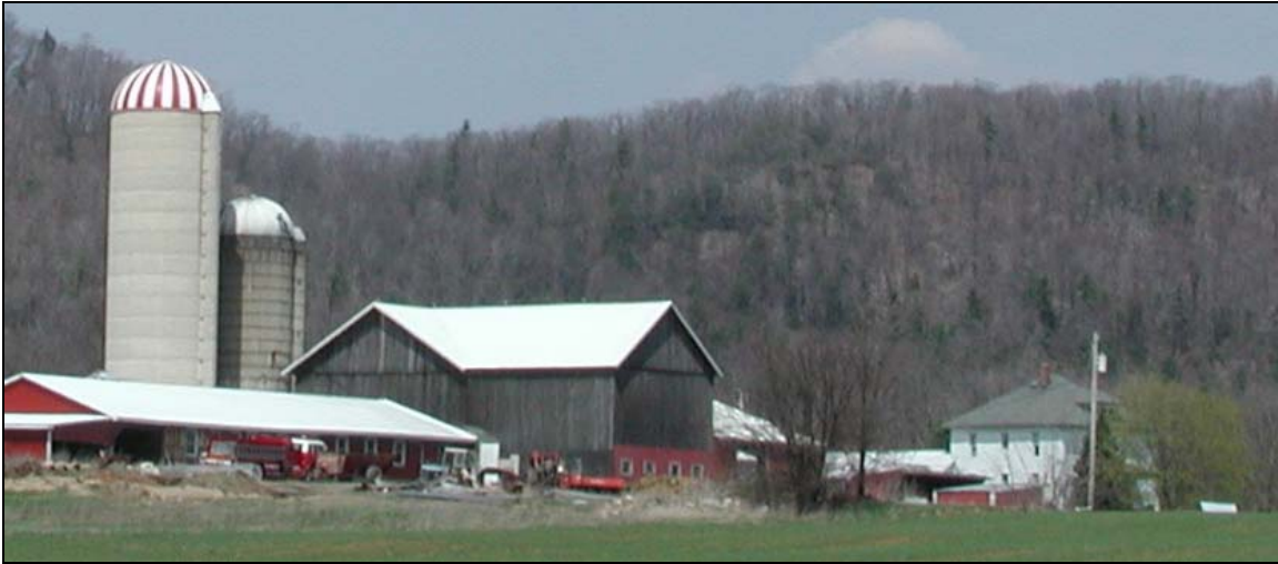
Black Hawk Road, Centre County. This picture illustrates some of the key changes of the 20 th century: poured concrete and concrete stave silos; three gable barn altered for dairy (note the windows cut into the lower level); pole barn (post war); foursquare house.
