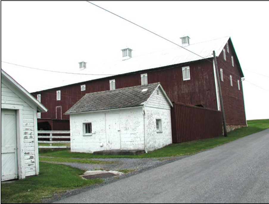
Concrete block milk house, Middle Road, Centre County.
