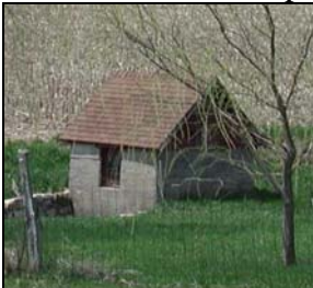
Spring house, Rhoneymeade, Harris Township, Centre County
