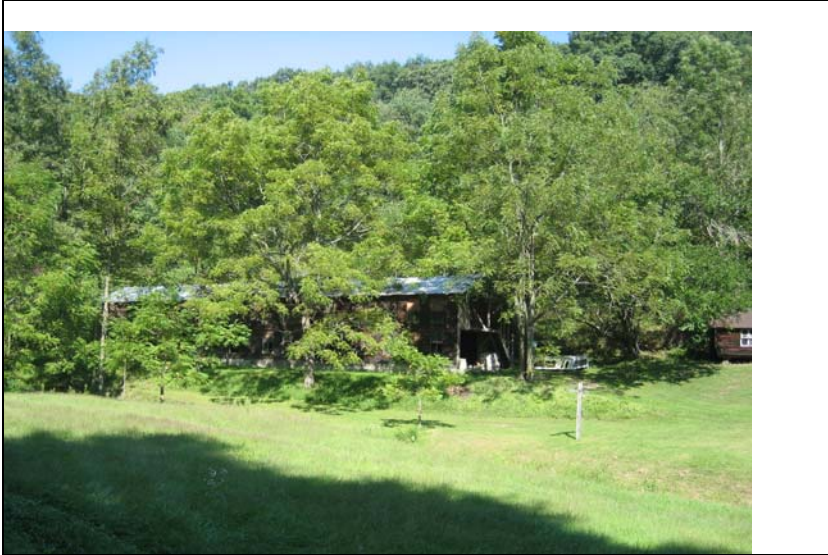
Multistory poultry house, Kellerville Road, Juniata County.
