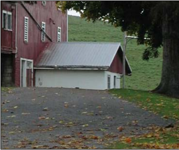
Milk house adjoining barn, at farm lane, Long Lane, Centre County.
