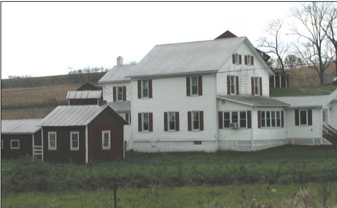
Summer kitchen in foreground, Paradise Road, Centre County.
