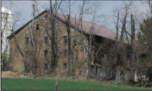
Neff stone end barn, Potter Township, Centre County.
