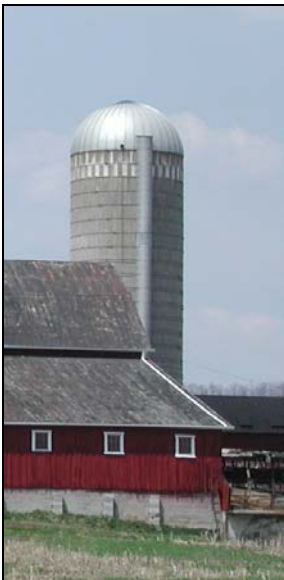
Concrete stave silo with hemisphere roof and metal chute, Rhoneymeade.
