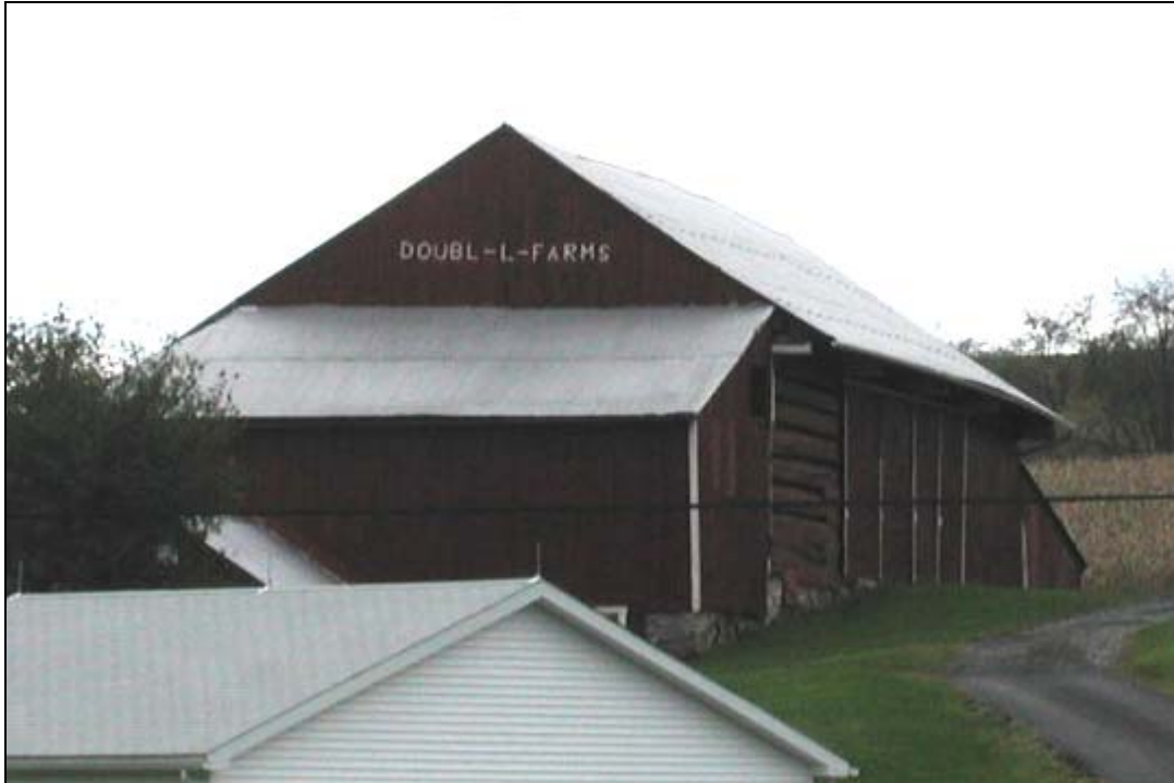
Double L Farm barn, Paradise Road, Centre County; shed roof corn crib on gable end of barn that is at least partially built of log.
