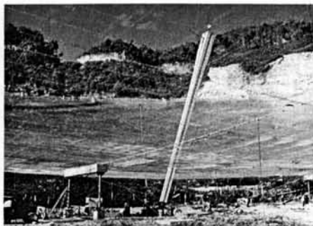
Fig. 35 August 14, 1963, the 430-MHz line feed is lifted.
