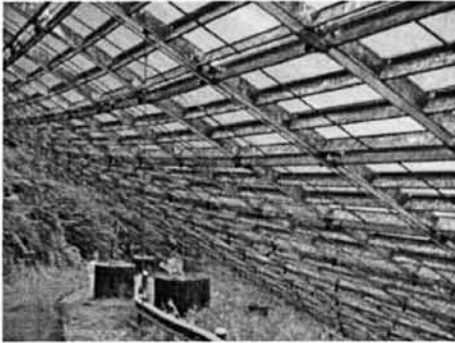
Fig. 39. Aluminum network that holds the "dish".
