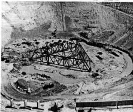
Fig. 33 Building the triangular platform in the ground, June 15, 1962.
