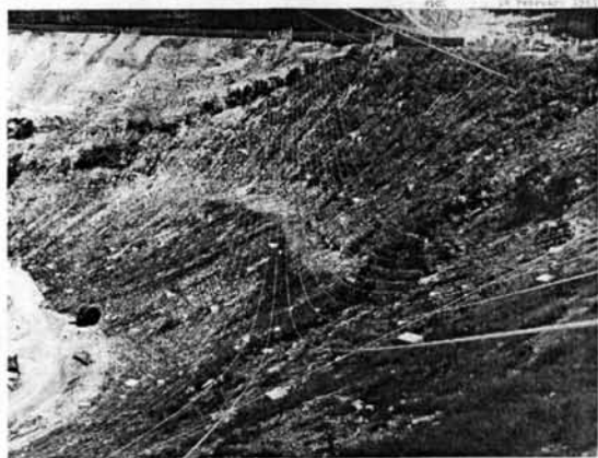
Fig. 36 Network of cables to hold the mesh layout, February 14, 1963.
