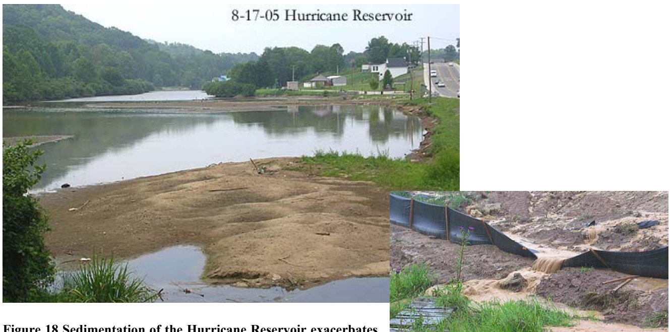
Figure 18 Sedimentation of the Hurricane Reservoir exacerbates low flow conditions and rapid flooding
