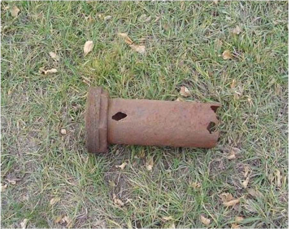
Figure 2. Corroded municipal water line from the town of Belt.
