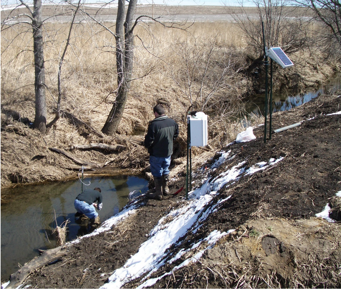
Fig. 3. Installation of Clear Creek monitoring station
