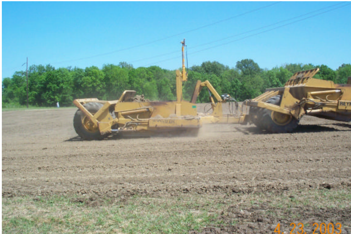
Figure 1. Laser-Guided Landforming at MS Runoff Field Site (ca. 3 Ac in size).
