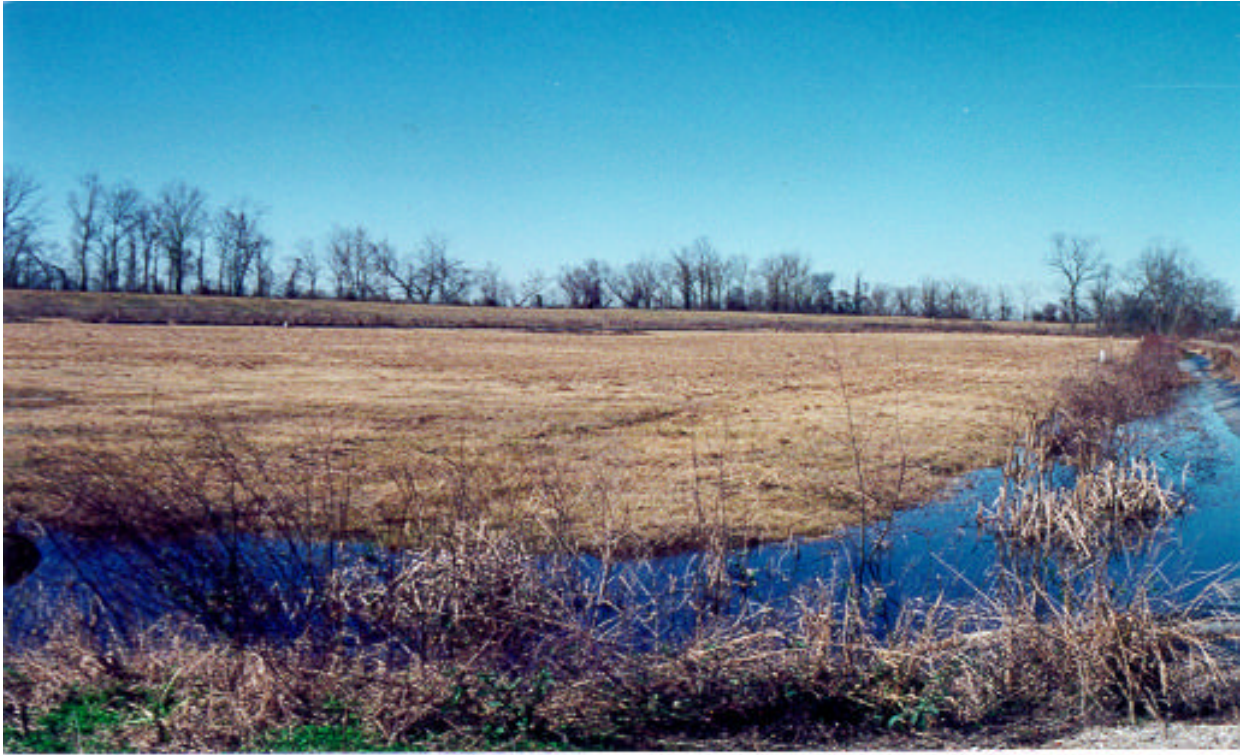
Land Treatment or bioremediation unit constructed during the Remedial Action, Phase I. (1990 - 1992)
