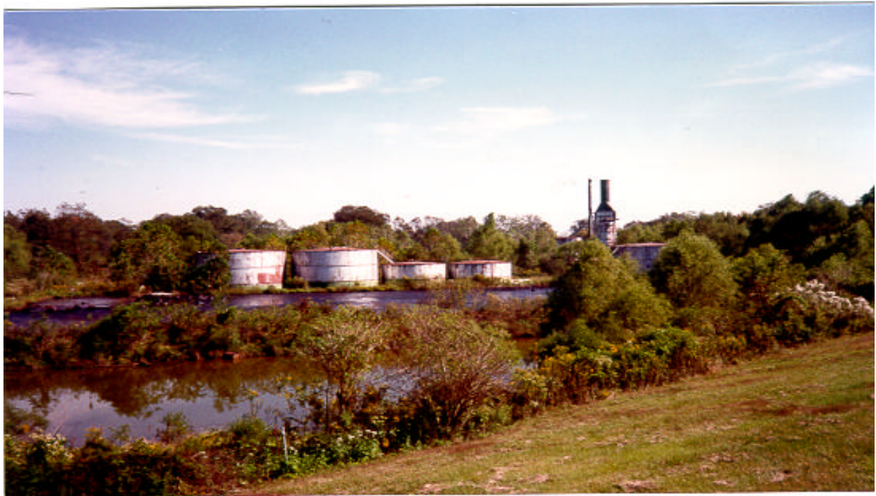
Both photos show on-site conditions before the start of the Remedial Action, Phase I, in 1990. Abandoned tanks, structures and lagoons are seen. (February 1990)
