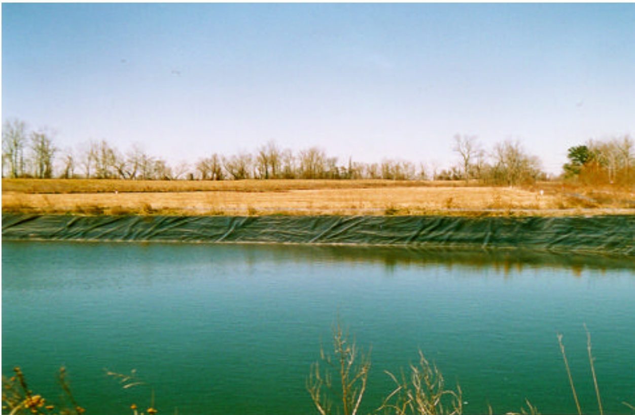
Lined impoundment constructed during the Remedial Action, Phase I. (1990-1992)
