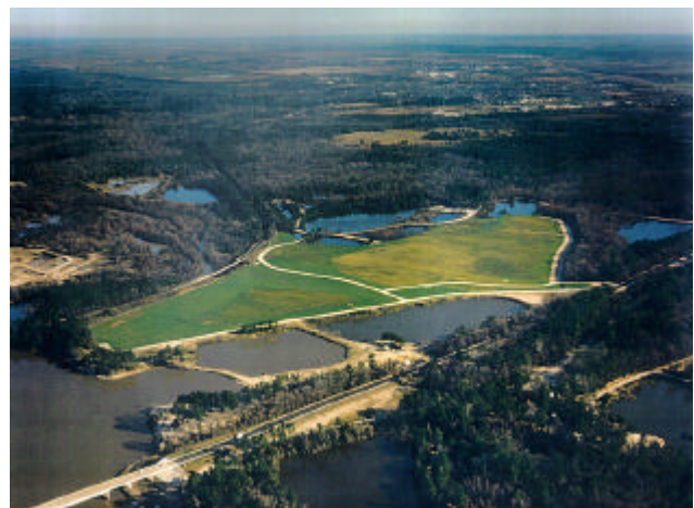
Completed condition - January 1995
