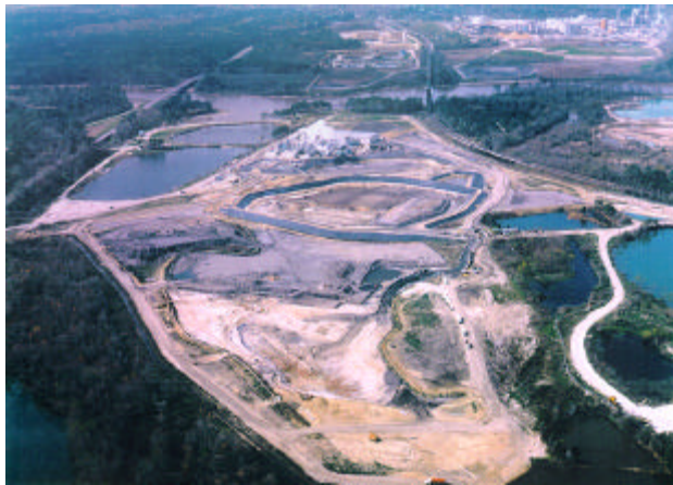
Phase B Construction and Remediation - March 1994
