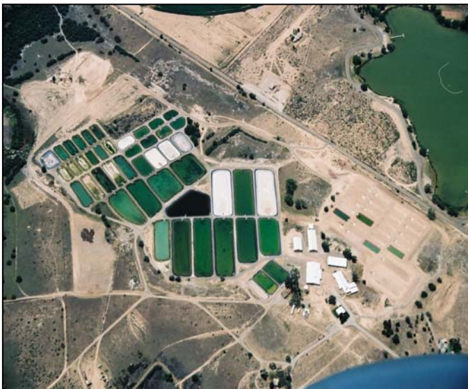
Ariel view of campus and facilities - Dexter, New Mexico
