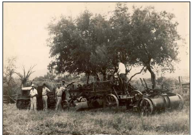
Beginning construction of Inks Dam NFH, May 1938
