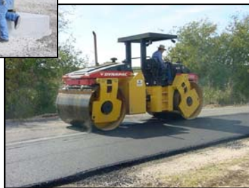
Constructing new state-of-the-art facilities
