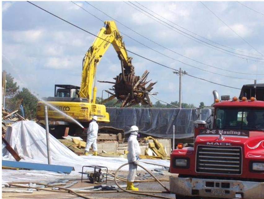
Figure 4. Transfer of building debris to truck bed.
