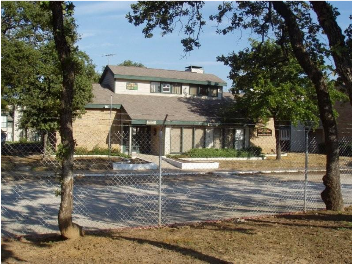
Figure 2. Oak Hollow Apartment Complex Office Building located at 5901 Boca Raton in Fort Worth, Texas.
