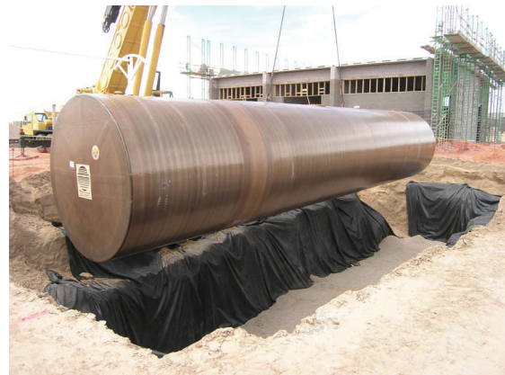
Installing a new underground storage tank at a facility
