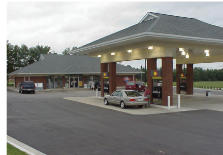
Underground storage tanks are located at gas stations and other non-retail locations
