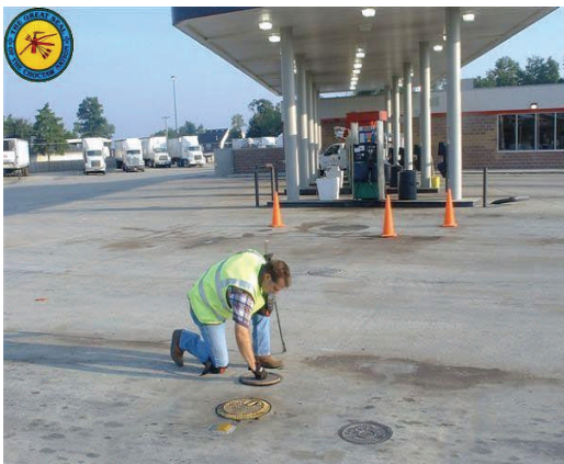
Inspecting a spill bucket
