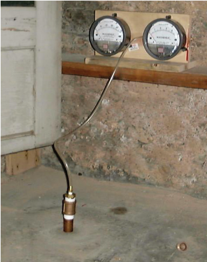
Figure 24. Magnehelic gauges and suction hole used for vacuum measurement.
