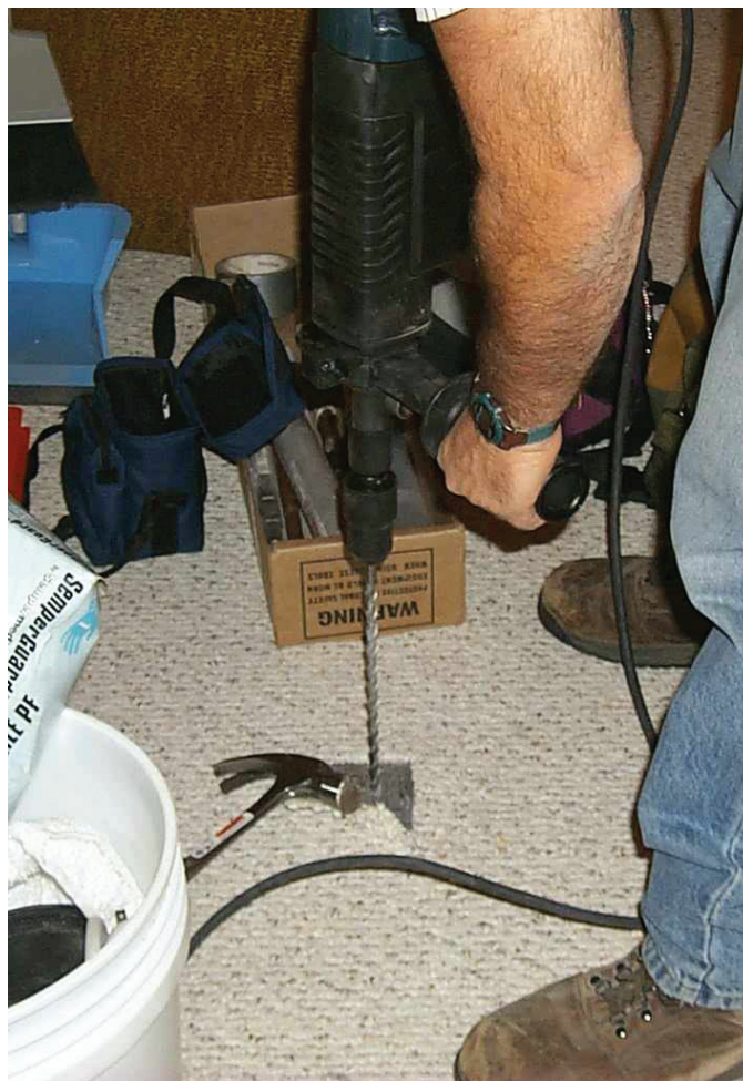
Figure 15. Drilling through a concrete slab using a rotary hammer drill.
