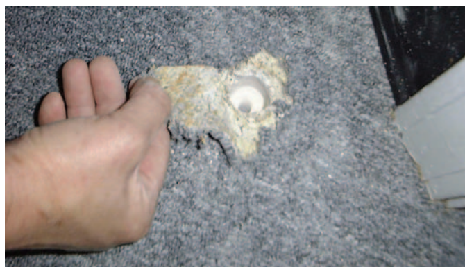
Figure 16. "Inner" and "outer" holes drilled in a concrete slab.
