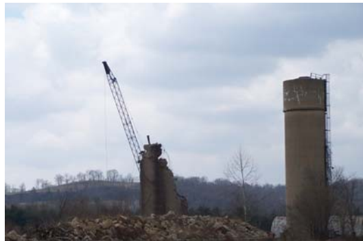
South Point Plant prior to remediation Source: EPA
