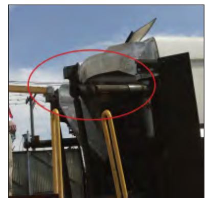
Talgo coach car tower support structure (circled). (Photos courtesy of Richard Clark of Raul V. Bravo & Associates, Inc., Reston, VA.)
