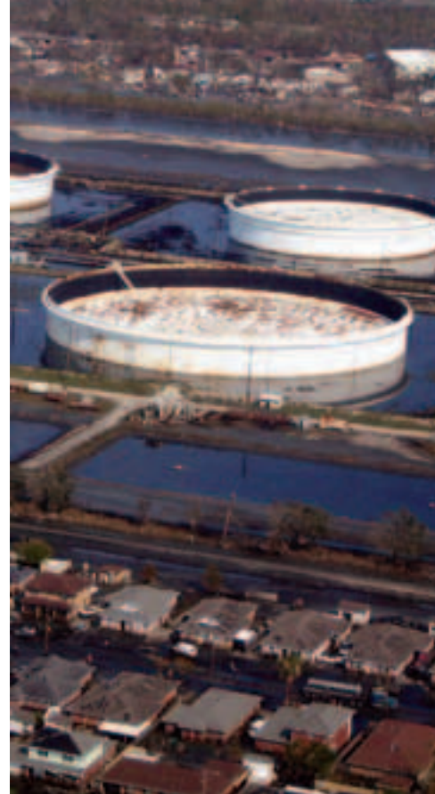
Murphy Oil refinery spill.
