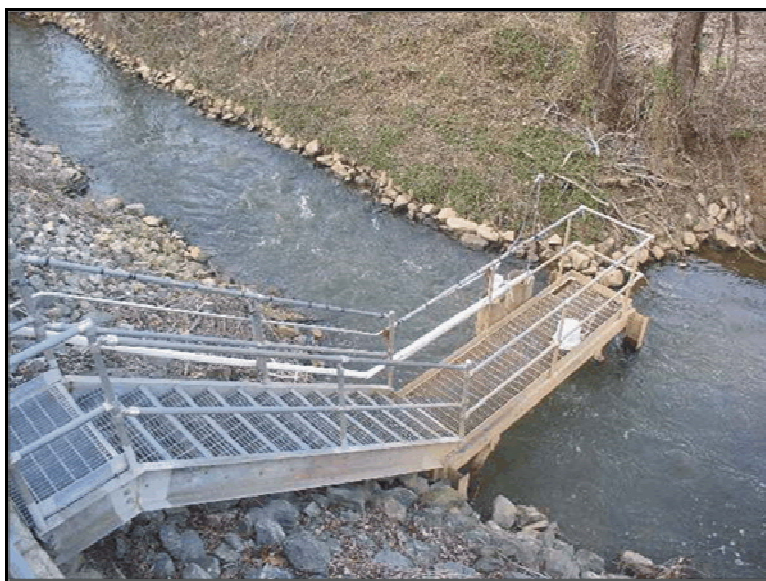
Figure 3-2. DuPont Spruance Final Effluent
