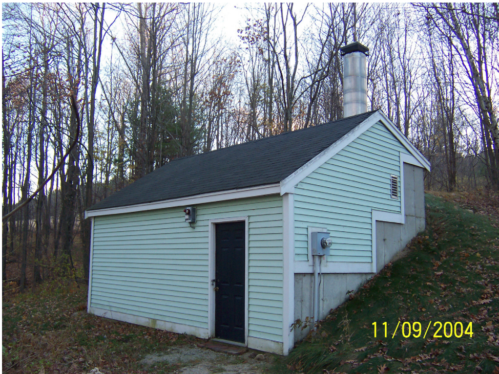
Figure 4-1. Preexisting Treatment Building at Orchard Highlands Subdivision
