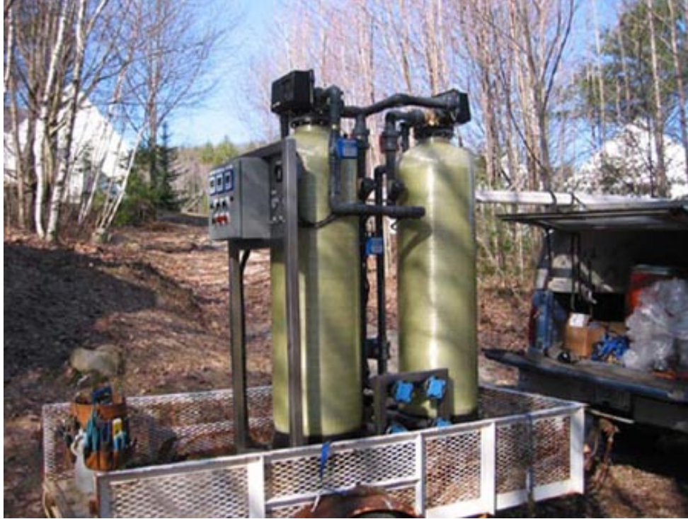
Figure 4-10. System Being Delivered to Site
