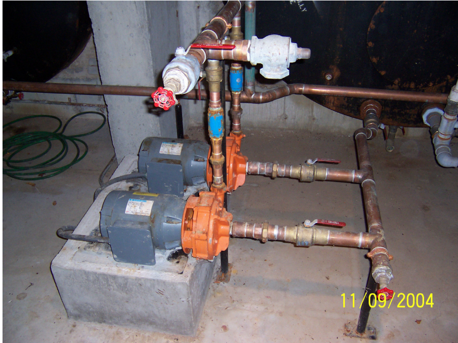
Figure 4-4. Booster Pumps
