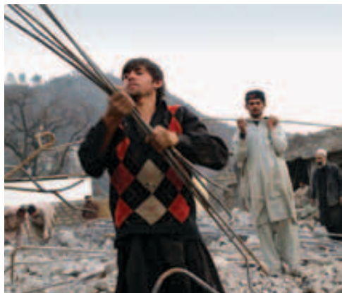
RECYCLING STEEL RODS: In Muzaffarabad, workmen salvage steel reinforcing rods from the rubble of buildings destroyed by the earthquake.
