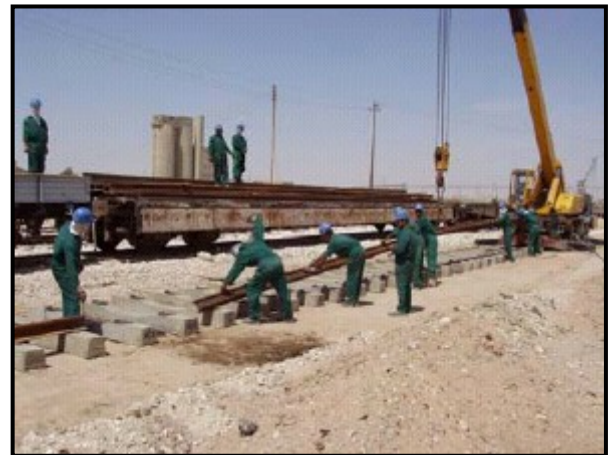
Laying track in southern Iraq
