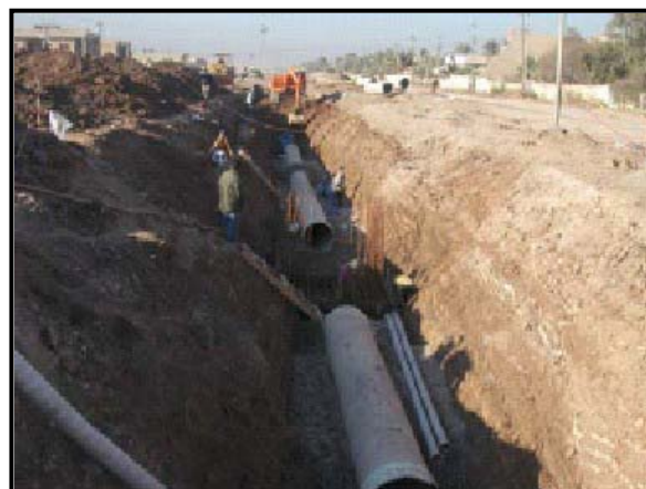
Workers install a new sewage line in Baghdad.
