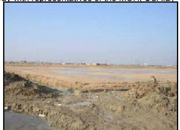
Ground being prepared for the children's hospital.
