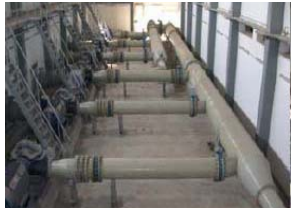
Expanding a water treatment plant in Baghdad.
