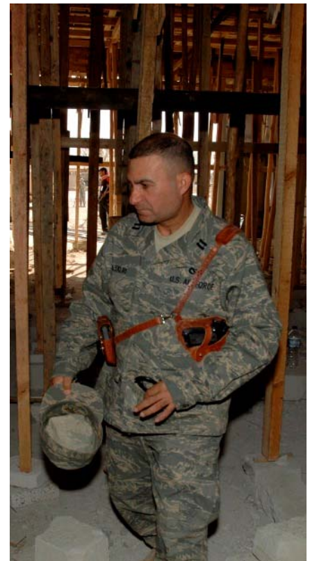
Captain Alsalih oversees a construction project in Iraq
