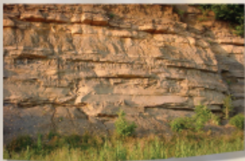
High wall from an old, abandoned strip mine.
