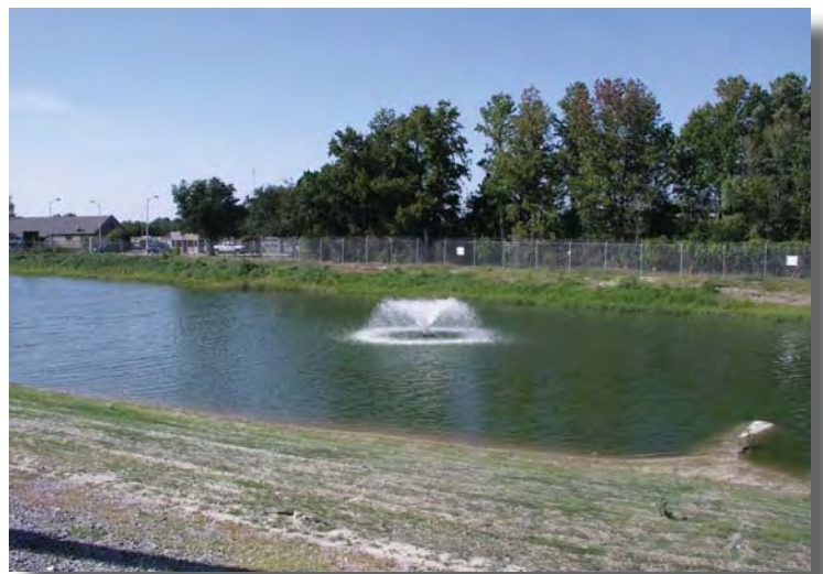
North pond of APM’s stormwater system also features aeration.
