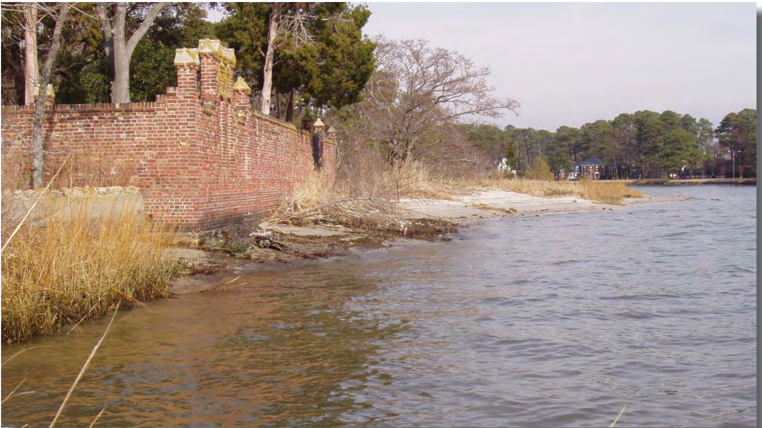
Before- A wetland at the Hermitage Museum in Norfolk, VA was eroding, threatening the historic wall and providing severely degraded habitat.
