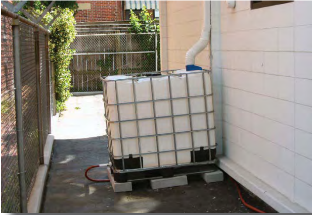
A plastic container is recycled to collect rain water at NOAA's Atlantic Marine Center in Norfolk. Rain barrels are a preventive measure not only for runoff pollution, but for water scarcity, an emerging global issue.
