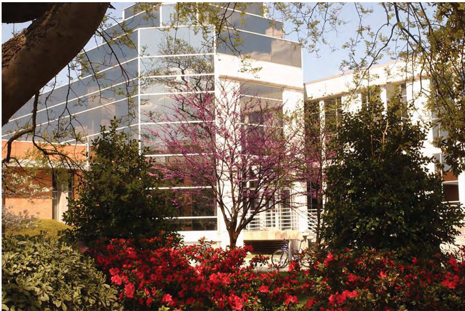
Old Dominion University built Virginia's first LEED (Leadership in Energy and Environmental Design) certified higher education building, housing Engineering and Computational Sciences. The building maximizes natural daylight. Office lights turn on and off by motion sensors.
