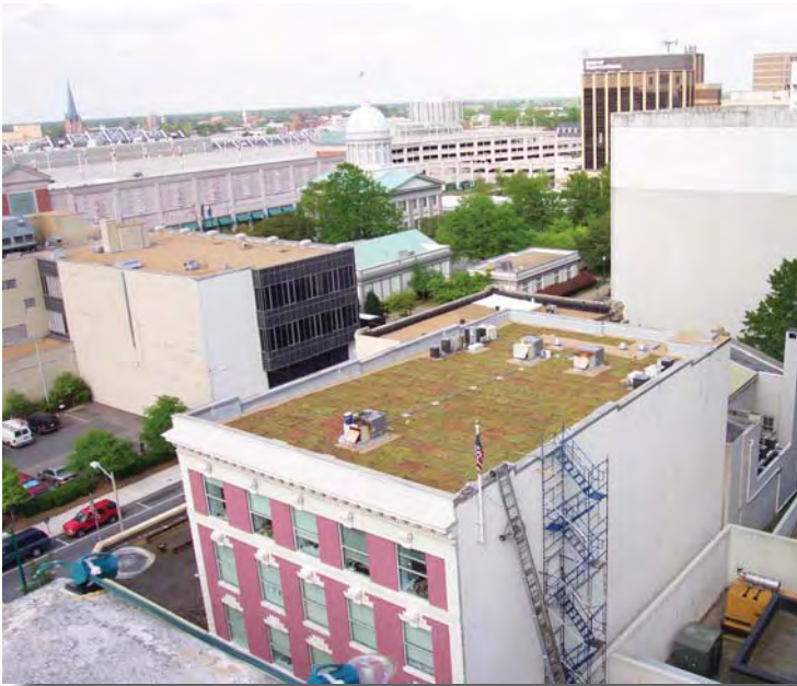
Atlantic Associates installed a green roof on its office building in downtown Norfolk.
