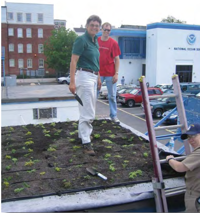
Succulent plants and engineered soils now filter runoff and extend the life of roofs on several of its smaller buildings at NOAA Marine Operations Center Atlantic in Norfolk, VA. Here, Pam Boatwright, River Stars program manager, and Doug Smith, NOAA work with volunteers on installation day.
