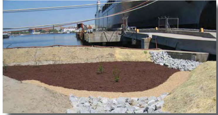
Retrofit in progress at Earl Industries.
