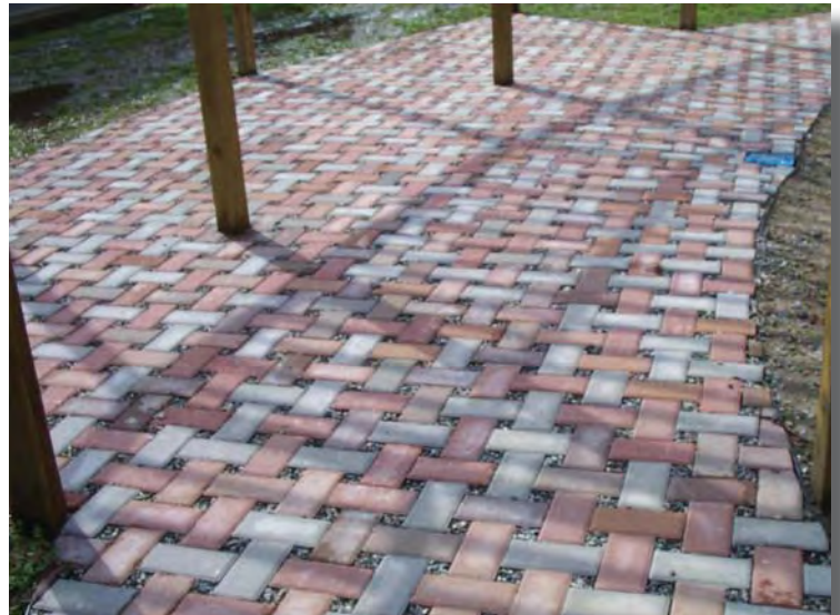
Norfolk Environmental Commission used volunteers to install this attractive pattern of bricks for its permeable, or rain-absorbing, sidewalks around the Ernie Morgan Environmental Action Center.
