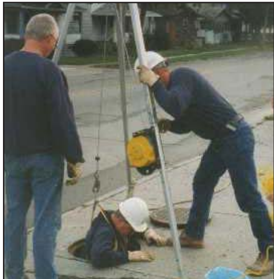
Trackdown sampling involves sampling water in local sewer systems for contaminants such as PCBs.
