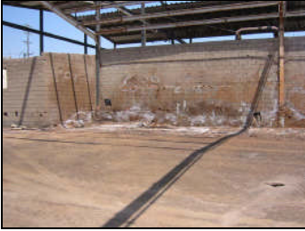
After Partial Clean Up (September 2004)
