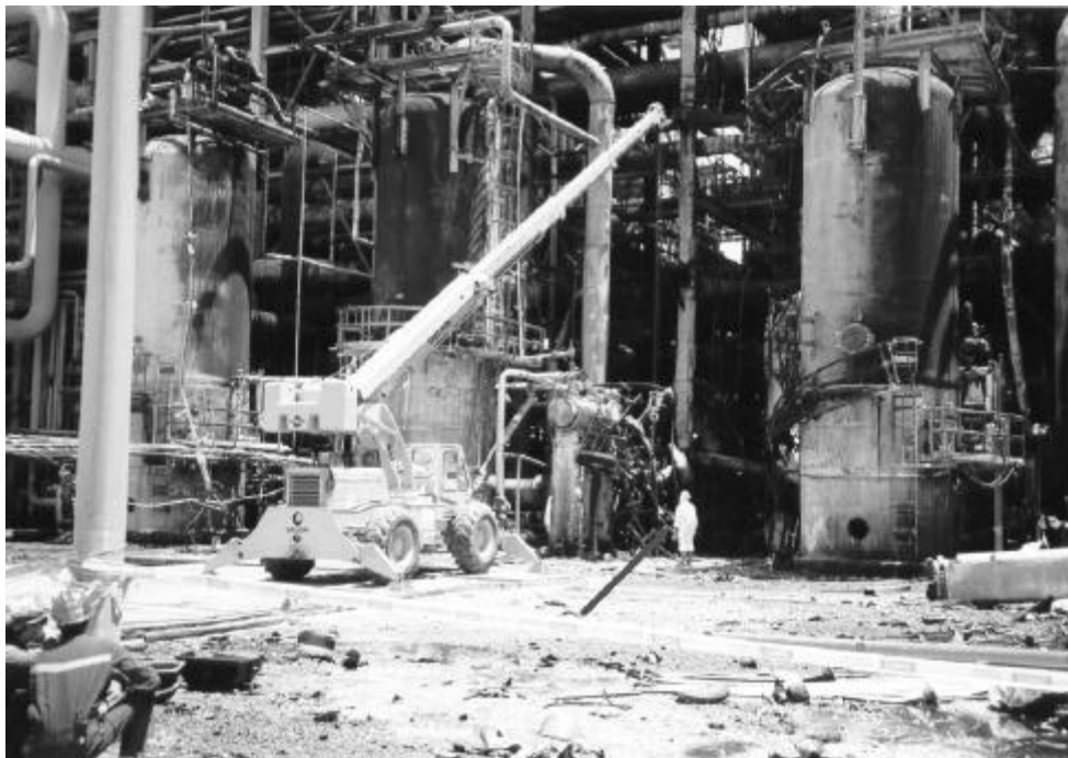
Figure E-6: Photograph of explosion and fire damage in the area of the PGC fifth stage suction and discharge drums (viewed from the north). The man in the lower center provides a reference to the scale of the surrounding structures. The failed check valve was located behind the drum to the man's right.
