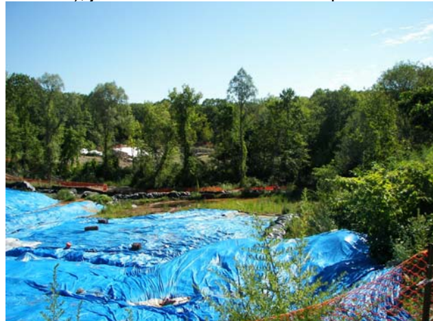
Figure 2. Removal activity at SR-3 (sludge removal area 3), just north of the O'Connor Disposal Area.
