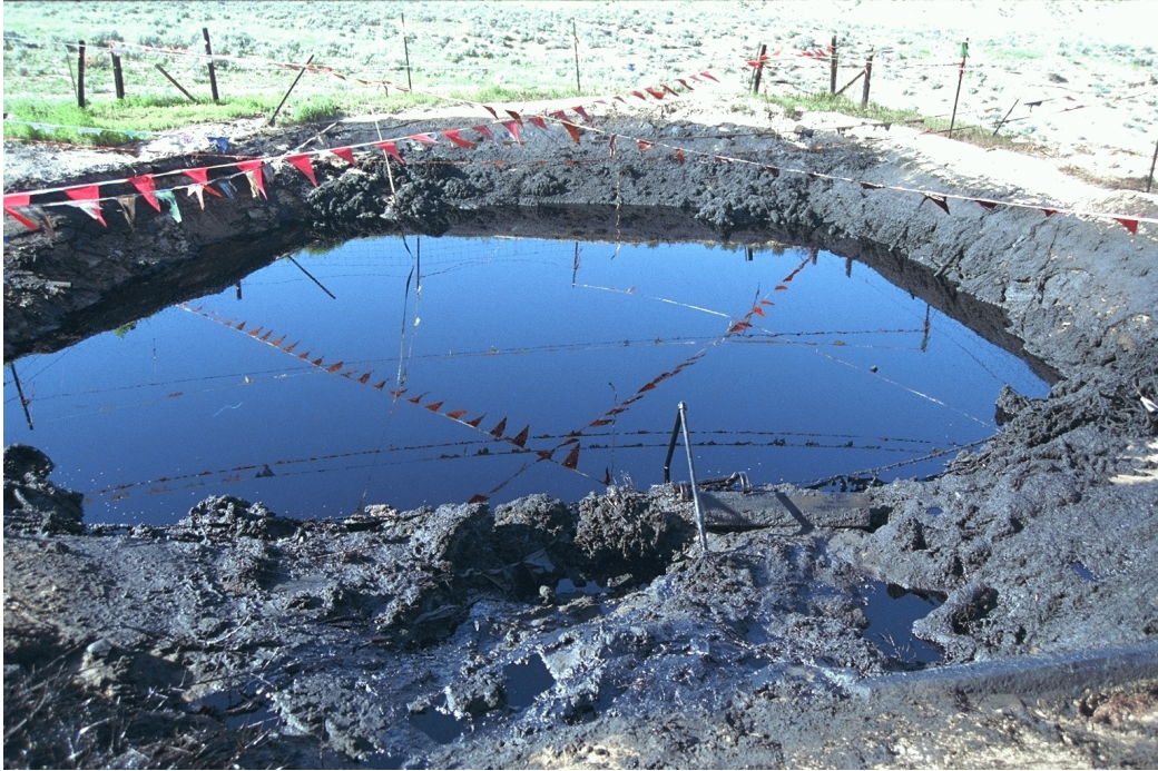
Figure 1. Oil covered pit with stained sides, evidence of overtopping of sides, and no effective wildlife exclusionary device.
