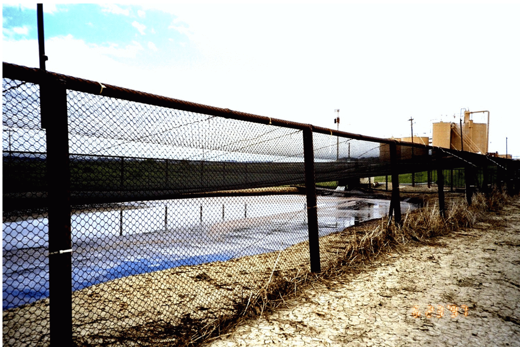
Figure 5. Photo of facility where netting has been installed as an effective exclusionary device to prevent birds and wildlife from entering pits which might contain oil.
