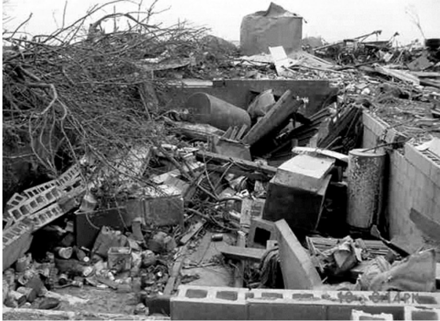
Fig. 3b. F4 damage to a farmstead in southwestern Barnes County, North Dakota, from the violent tornado. Photo by Mark Ewens.
