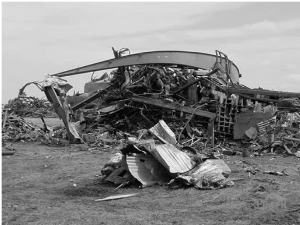
Fig. 3c. Debris pile from the violent tornado at the same farmstead as in Fig 3a. The bent steel I-beam on top indicates F4 damage. Photo by Mark Ewens.
