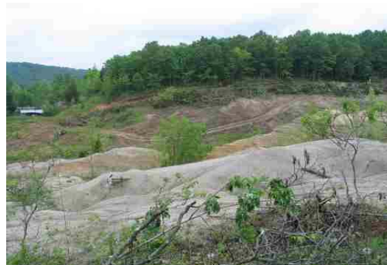
View of tailings and wind row of trees. Crews have to remove trees and construct roads before the tailings can be stabilized.
