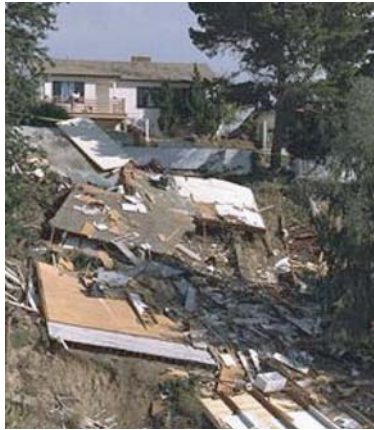
Landslides —Earthquakes can trigger landslides that damage roads, buildings, pipelines, and other infrastructure. Steeply sloping areas underlain by loose or soft rock are most susceptible to earthquake-induced landslides. This home was destroyed when the hillside beneath it gave way following the 1994 magnitude 6.7 Northridge earthquake (FEMA photo).
