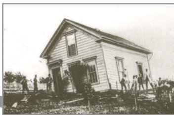
1868—Damage in Hayward
