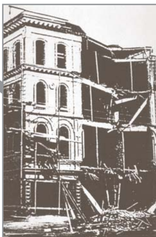
1865—Damage in San Francisco
