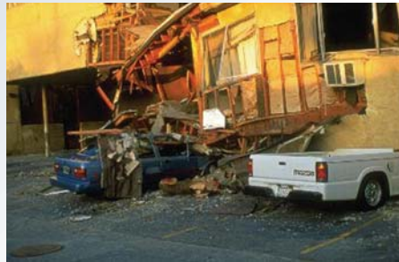
The “soft” first story of this apartment building collapsed in the 1994 magnitude 6.7 Northridge earthquake, crushing cars below and severely damaging the floors above (FEMA photo).
