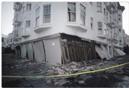
Buildings in the Marina District of San Francisco were badly damaged in the 1989 Loma Prieta earthquake. “Soft story” buildings, typically with parking on ground floor, like the one pictured here, are common throughout the Bay Area and are particularly at risk when exposed to strong shaking. (USGS photo)
