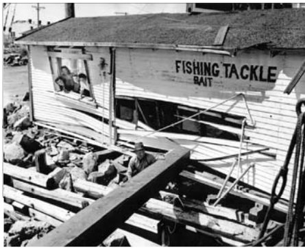
Tsunamis —Great earthquakes occurring anywhere in the Pacific Ocean may displace the ocean floor, generating tsunamis that could affect the California coast. Some coastal communities are designating Tsunami Hazard Zones and planning evacuation routes. Although the tsunami hazard in most of the Bay Area is low, coastal areas are still at risk. For example, this bait shop (Hazel's Fish Stand) in Half Moon Bay was ruined when it was hit by debris in the tsunami generated by the 1946 (magnitude 8) Alaska earthquake (photo copyright by MS & SB Collection).
