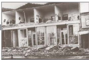
1906—Damage in Healdsburg
