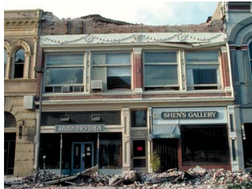
These small businesses in Santa Cruz, California, were heavily damaged in the 1989 magnitude 6.9 Loma Prieta earthquake, but both eventually reopened (USGS photo).
