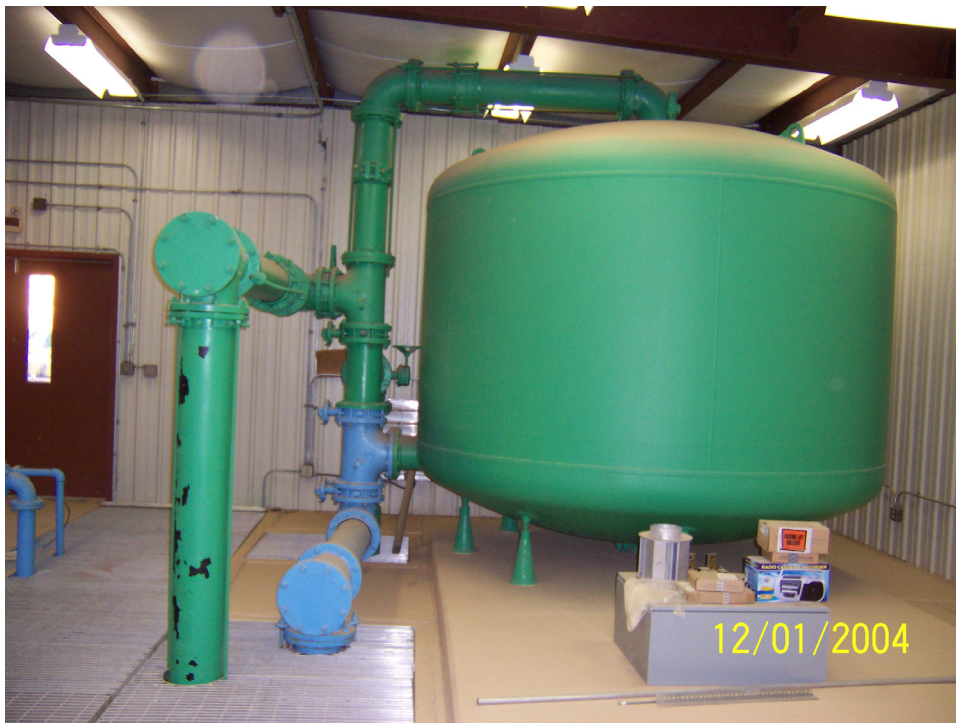
Figure 4-4. Inside of Preexisting Water Treatment Building with Unused Sand Filtration Vessel
