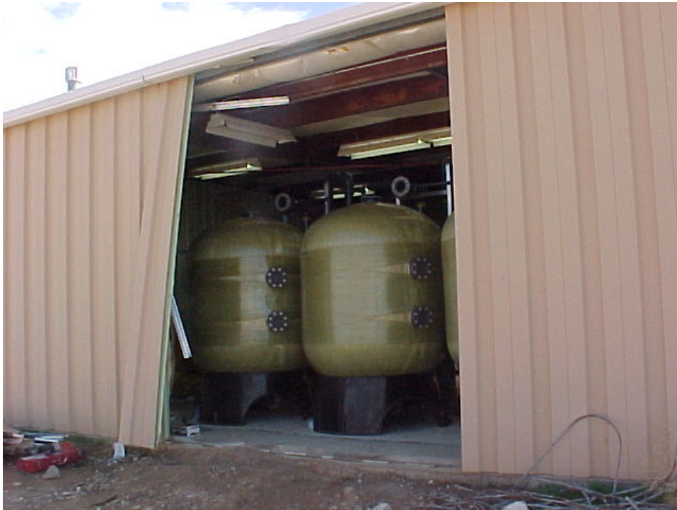
Figure 4-15. Removal of Treatment Building Side Wall Panel for APU-450 System Off-loading
