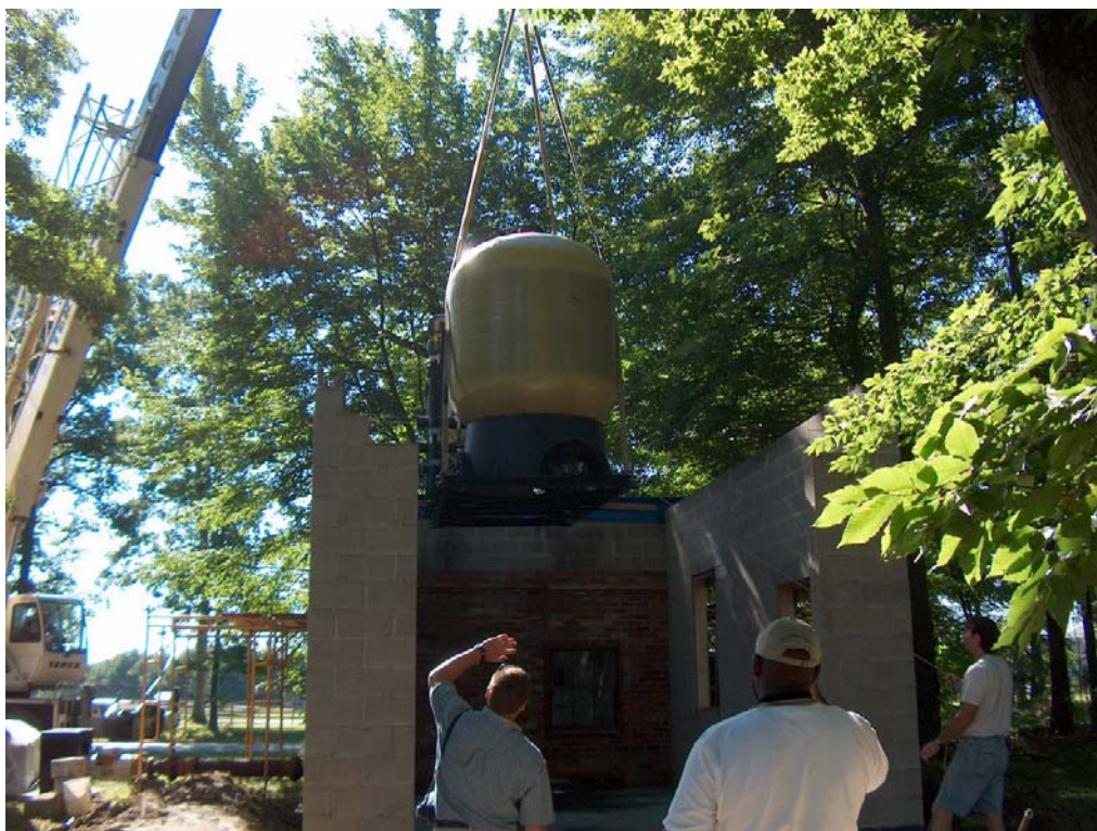
Figure 4-7. Unloading of APU Skid into Partially Completed Treatment Building Addition
