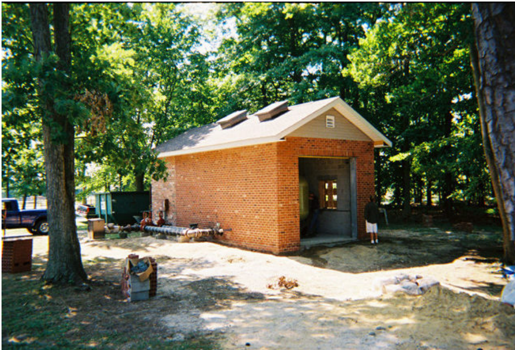
Figure 4-6. New Treatment Building Addition with Two Access Hatches on Roof
