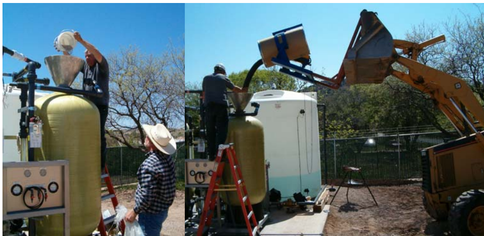
Figure 4-5. Gravel Underbedding (Left) and AD-33™ Media (Right) Loading
