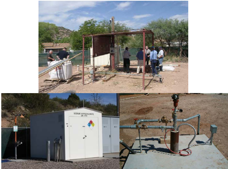
Figure 4-1. Predemonstration Site Photographs (Clockwise from Top: Condition in July 2003; Well No. 2 Wellhead after Redevelopment; and Chlorine Shed and Emergency Shower Station)
