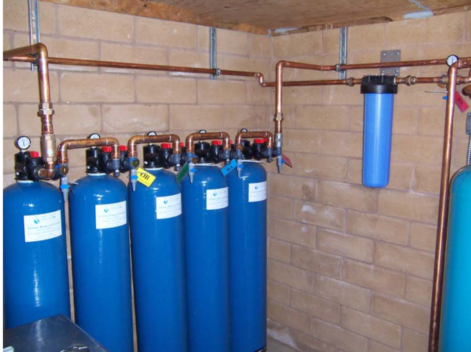
Figure 4-5. As/1200CS System with Oxidation and Adsorption Columns Shown Against Wall and a Sediment Filter Attached to Wall
