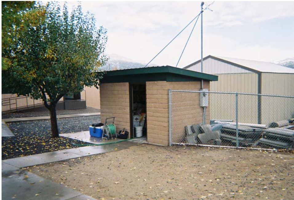
Figure 4-1. Pre-Existing Well No. 2 Pump House at Richmond Elementary School
