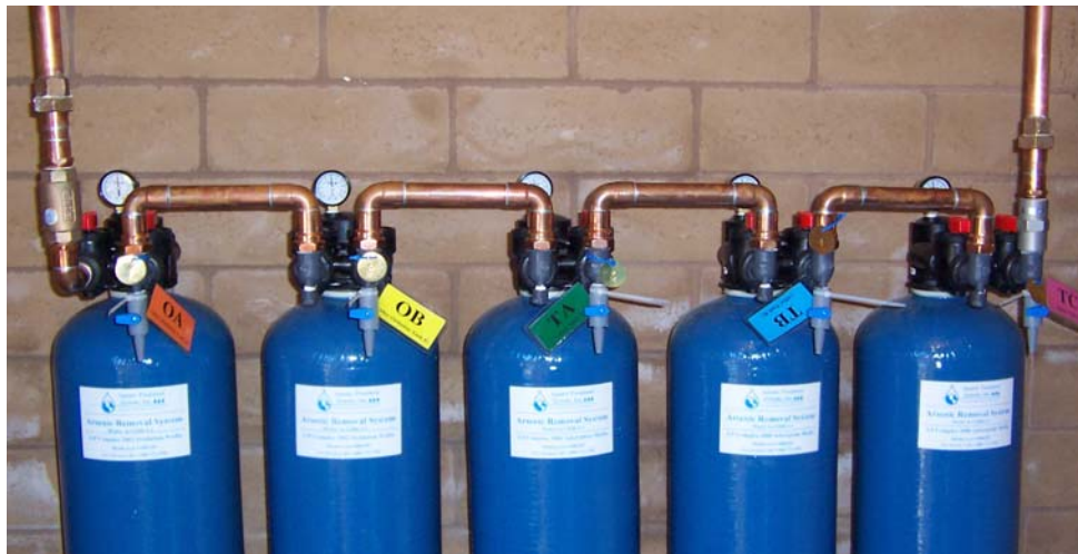
Figure 4-6. Close-up View of Oxidation and Adsorption Columns with Sample Taps and Labels
