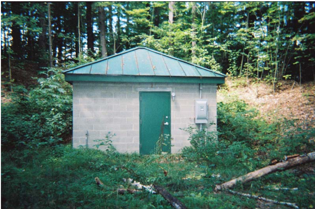
Figure 4-1. Pre-Existing Treatment Building at Charette Mobile Home Park
