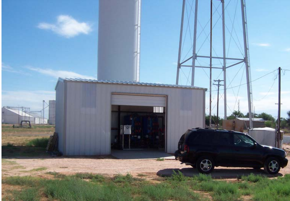
Figure 4-4. Water Treatment Facility in Wellman, TX
