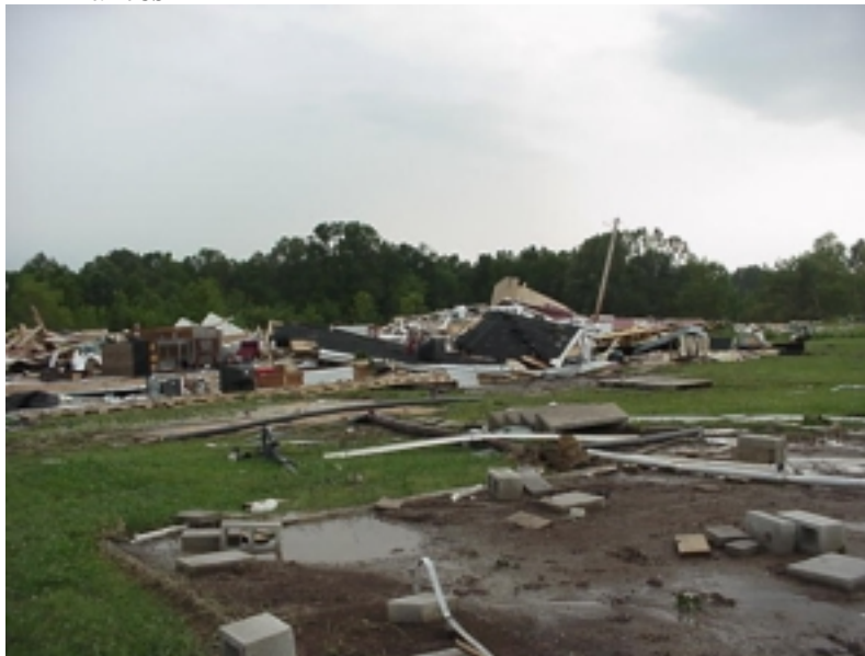
Several mobile homes were destroyed in Monroe County from a tornado which struck on May 7th. The tornado moved into Monroe County from Chickasaw County and continued to move east-southeast. A cow and a calf were killed. Thirty-five homes were destroyed and 117 others were damaged. Several barns, sheds and outbuildings were also damaged.
