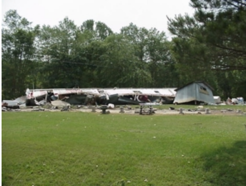
Damage at a trailer park in Lee County from a tornado that struck on May 6th.
